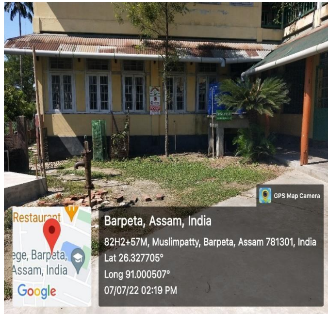
Figure 8: Rain water harvesting unit
