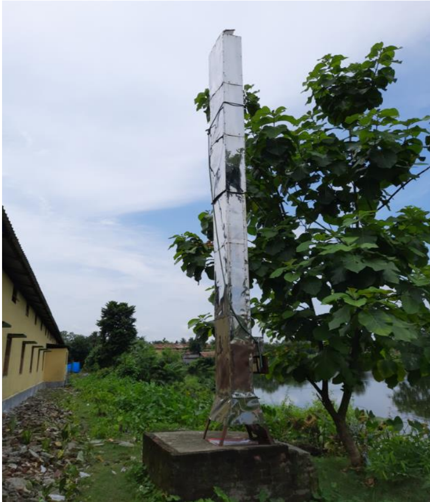
Solid waste disposal plant (chimney)
